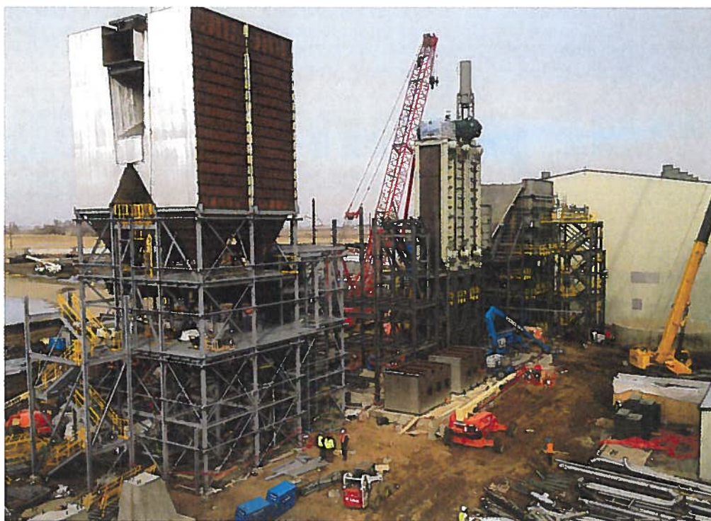
The Poet-DSM plant under construction in Emmetsburg, Iowa
